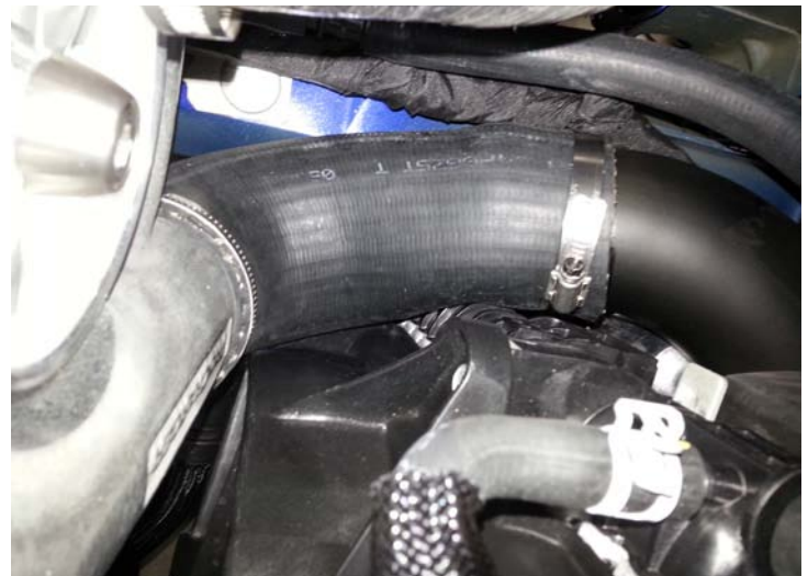
Blower Discharge Tube Installed
