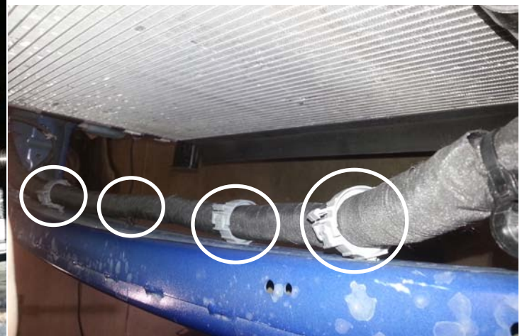
Wiring Harness Retainers
